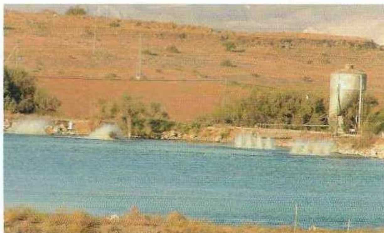
Figure 10.1: Aerators placed in one location in the pond 1
