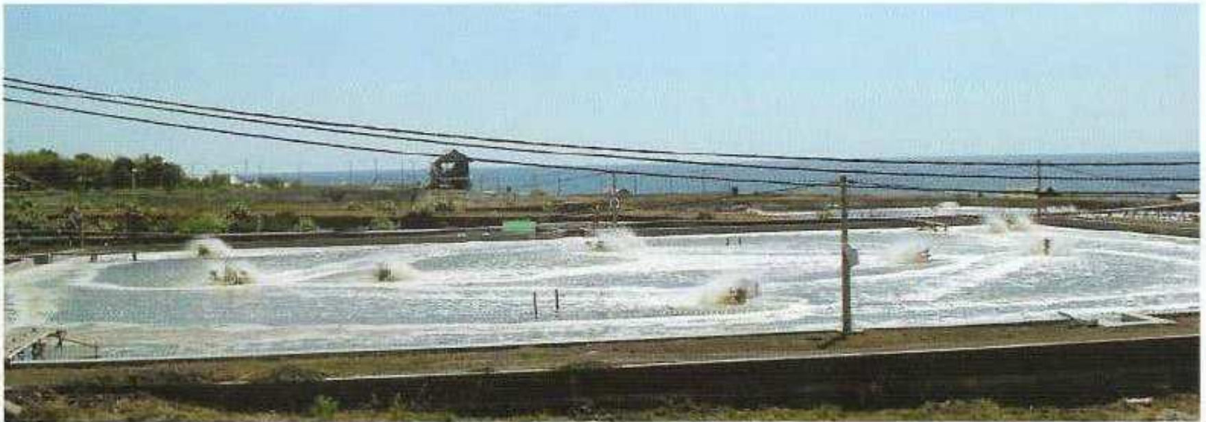
Figure 13.5: Aeration using two rings of aerators and aerators aimed at the center zone of the pond
