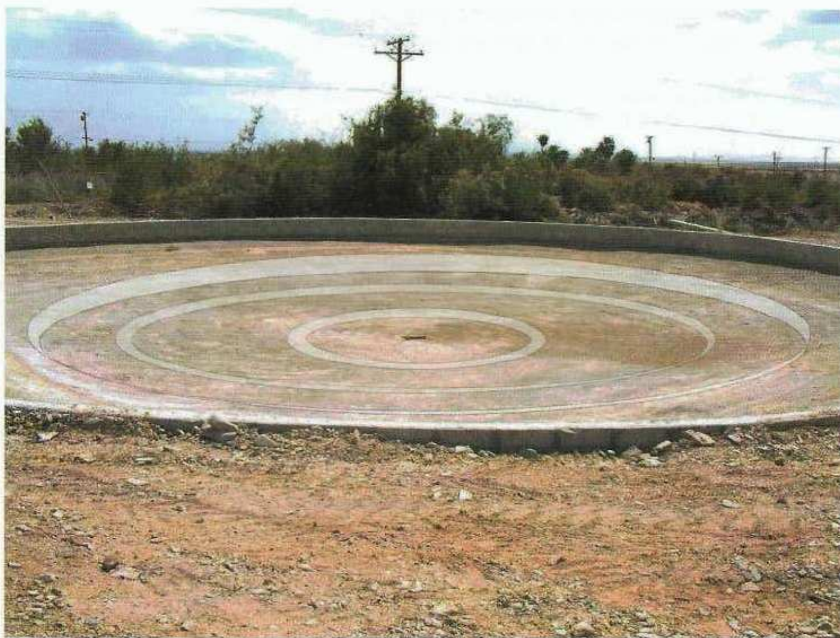
Figure 12.6: Pond slopping toward the drainage point
